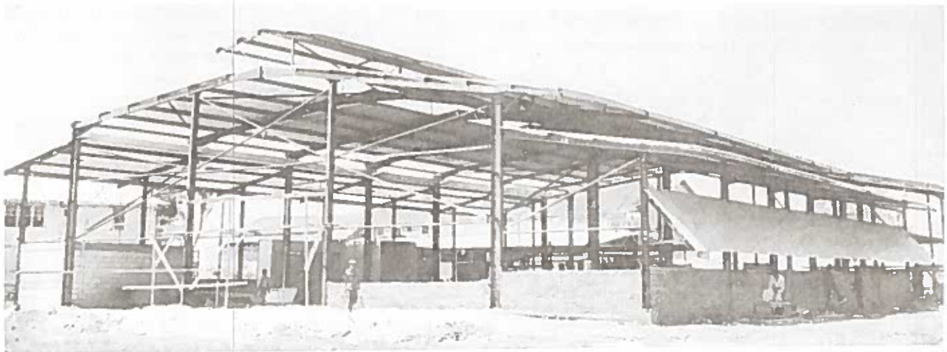
Equipment Conservation Centre under construction at Ogle.
