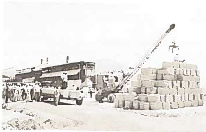
Compressed bagasse being conveyed for stacking.
