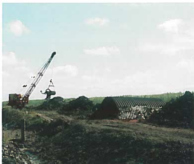
Bridges of the future: corrugated tubes being set in place
