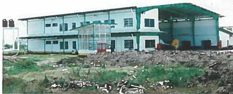
New hangar under construction at Ogle.
