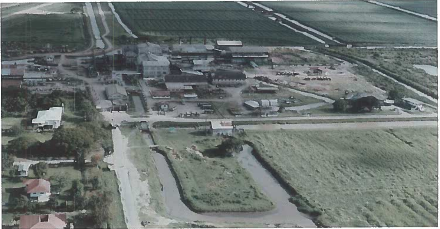
An aerial view of GUYSUCO's largest estate, Albion, which, together with Rose Hall Estate form the East Berbice Estate in keeping with the Board's new 5-year Strategic plan to boost production and all - round efficiency.
