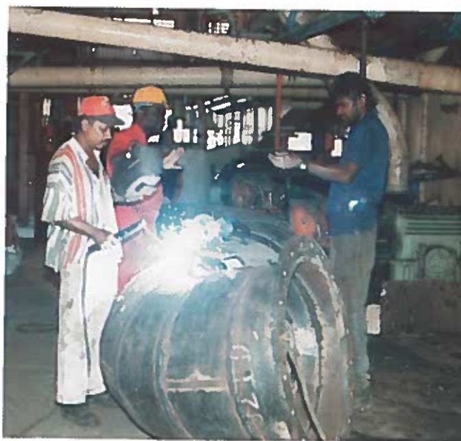
Cleaning of Juice Pipes
