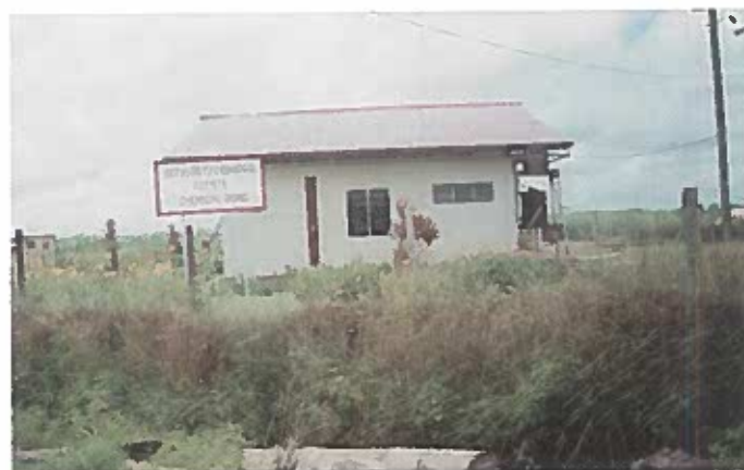
The bond at Uitvlugt Estate where chemicals for the industry are safely stored far away from other activities and personnel of that location.
