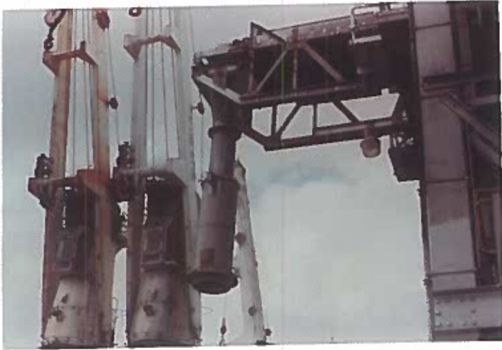
Sugar Terminals- Rehabilitation Work
