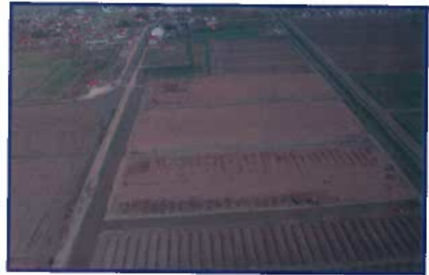
Aerial view of land preparation at the Skeldon Sugar Modernisation Project.
