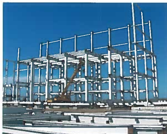
Process House under Construction
