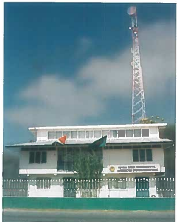
Communication Tower at ISD, Camp Street
