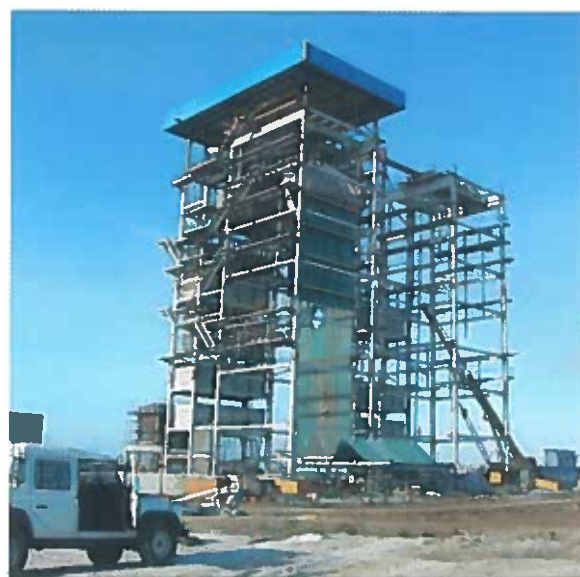
Steam Boilers under Construction
