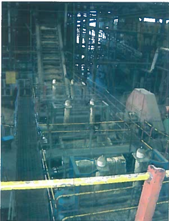
Factory Operations - Milling Train
