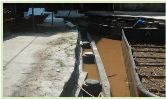
Milldock revetment at Albion
