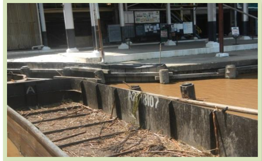
Milldock revetment at Albion
