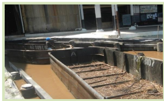
Milldock revetment at Albion
