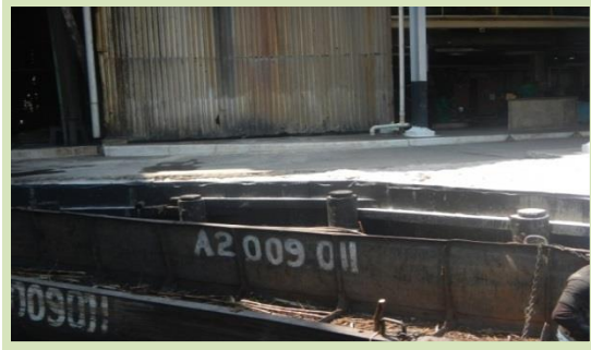
Milldock revetment at Albion
