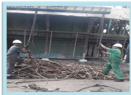
Cane Gantry Operation
