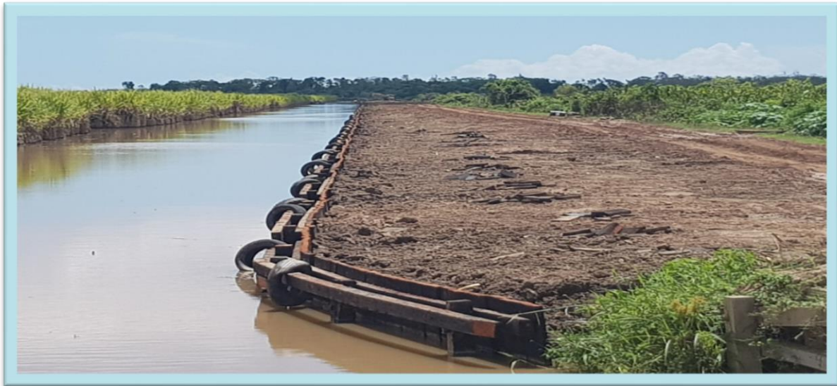
Revetment at Blairmont
