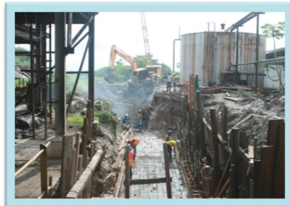
Blairmont Water Intake Channel Phase 2
