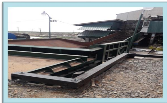
Billet Cane Conveyor at Albion
