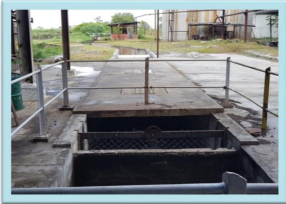
Blairmont Water Intake Channel - Completed
