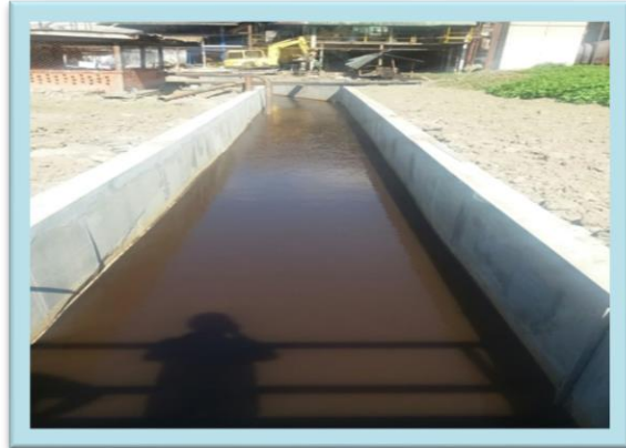
Blairmont Water Intake Channel - Completed
