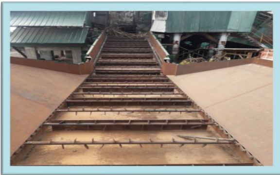
Billet Cane Conveyor at Albion
